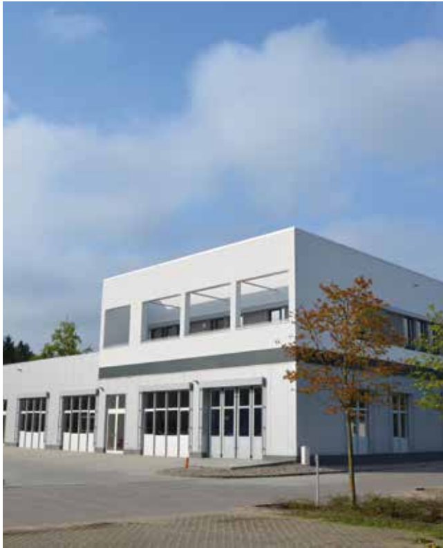
The incoatec headquarter
